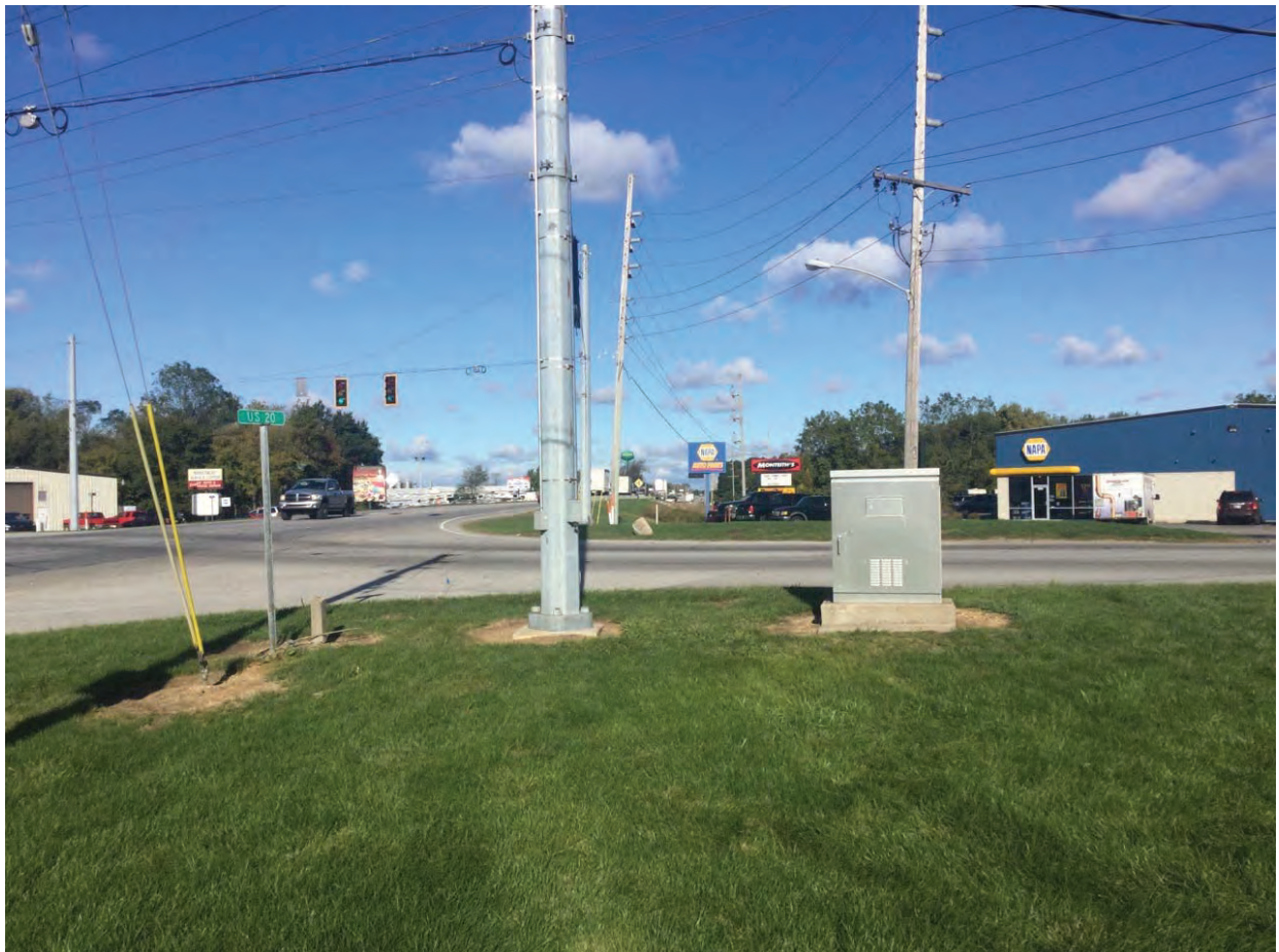
34. Looking north west along roadside US 20
