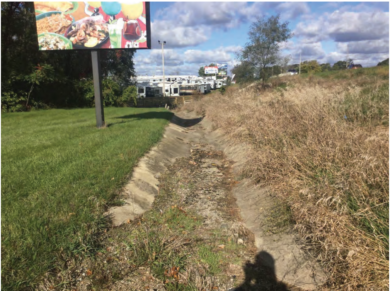
60. Looking north west that concrete side ditch
