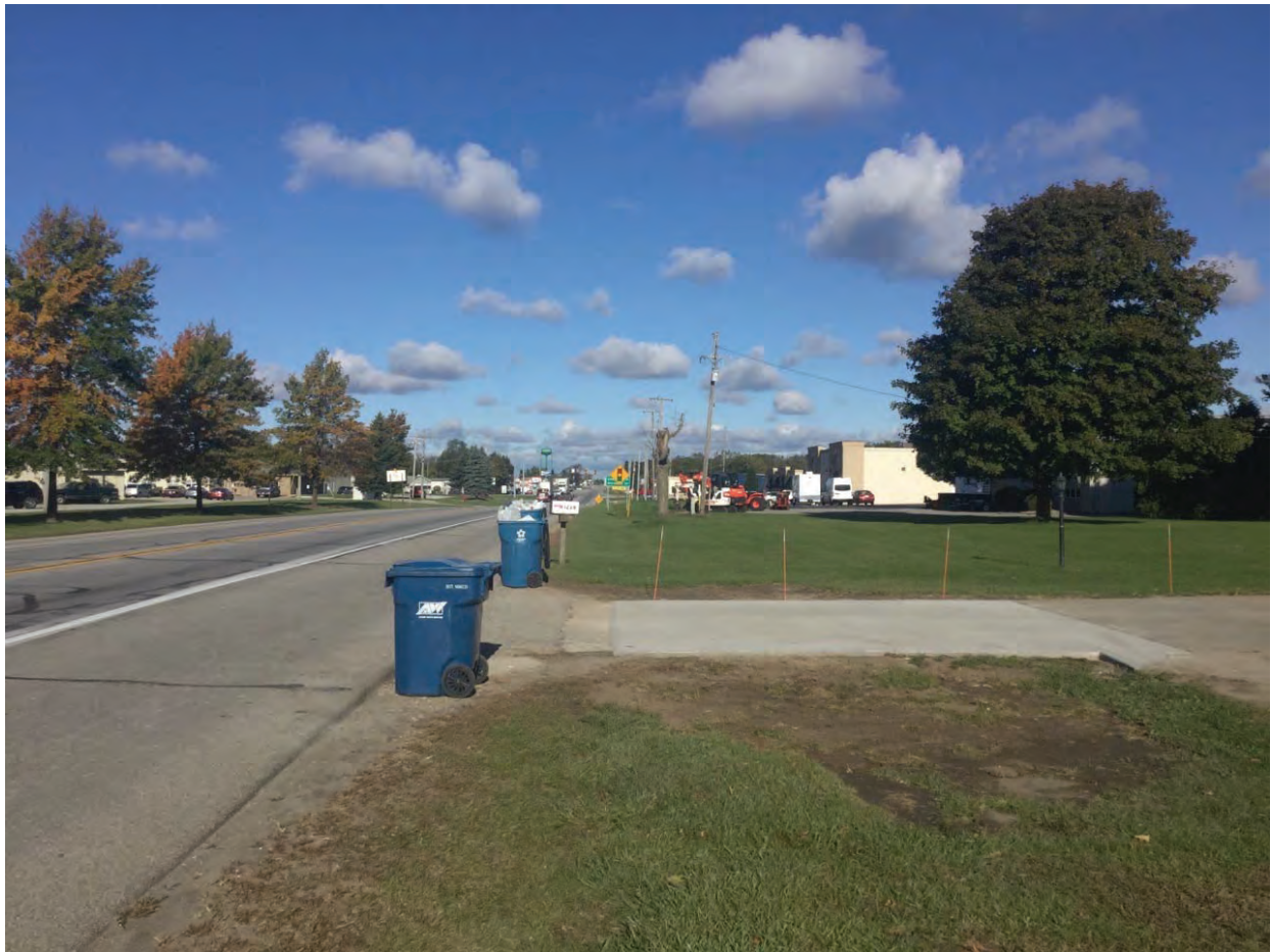
37. Looking north west along roadside US 20
