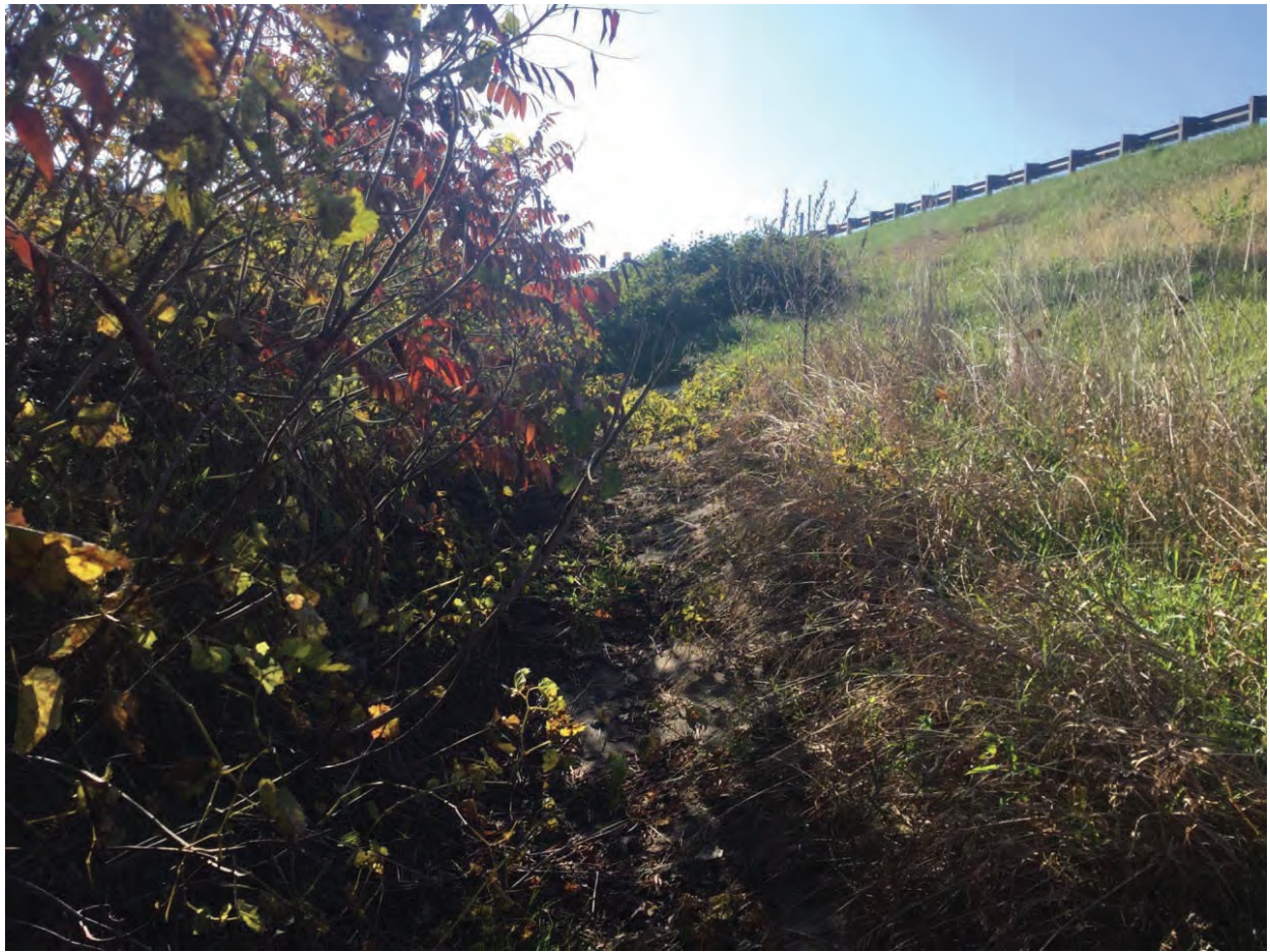
27. Looking south east up concrete side ditch
