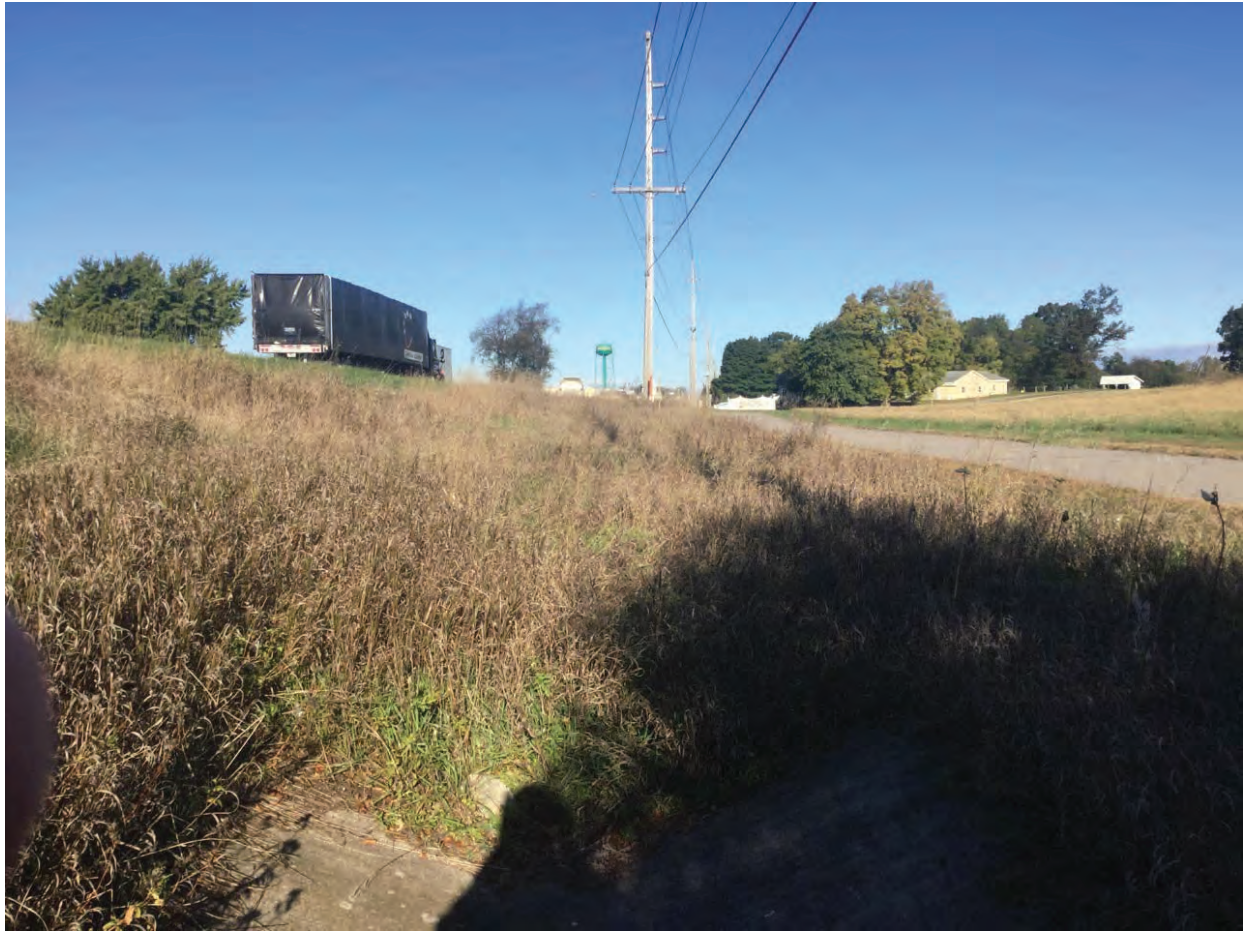
23. Looking north west along concrete side ditch
