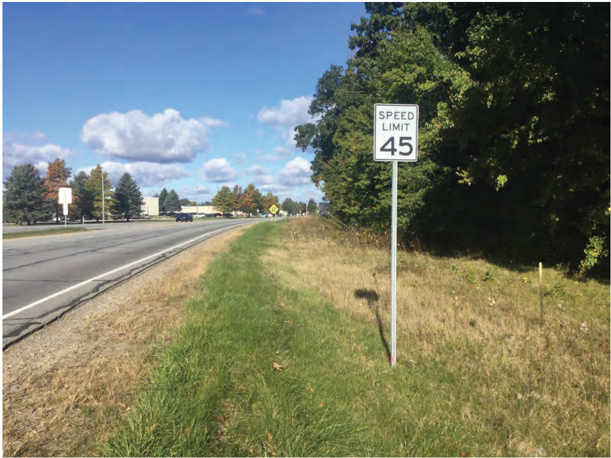
39. Looking north west along roadside US 20
