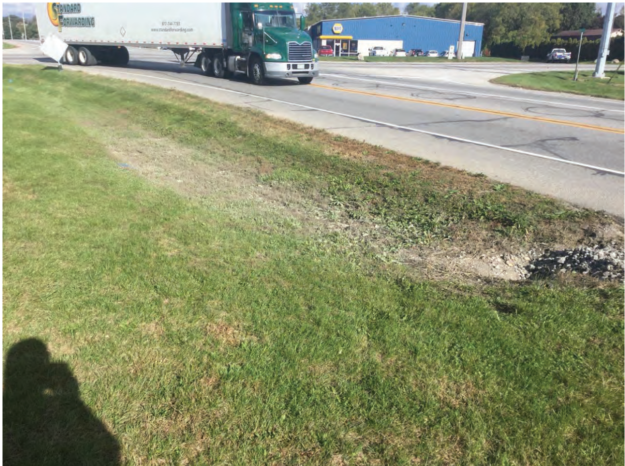
58. Looking north at roadside drainage area
