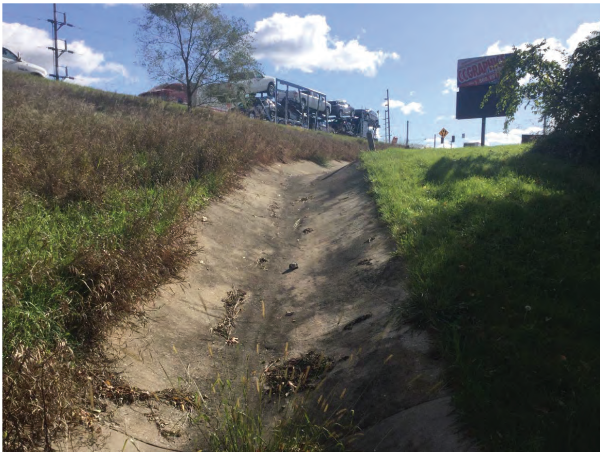
64. Looking south east at concrete side ditch
