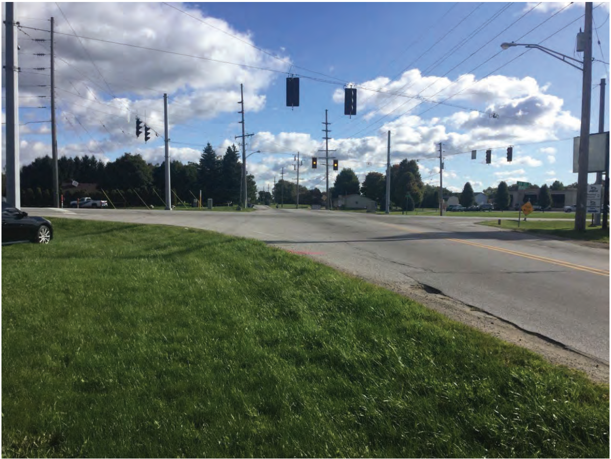
59. Looking north east at US 20 / CR 22 intersection
