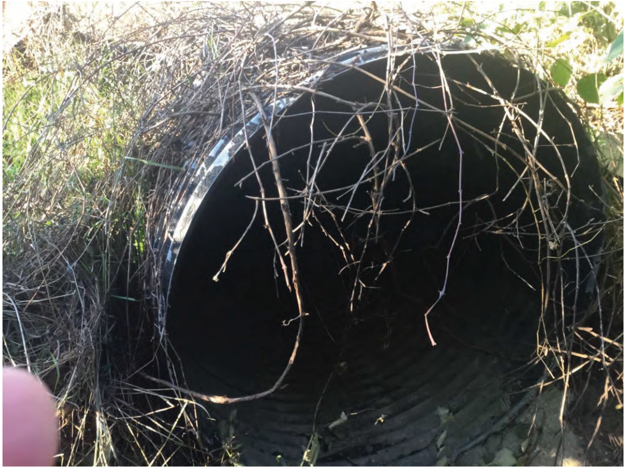
29. Looking west at culvert
