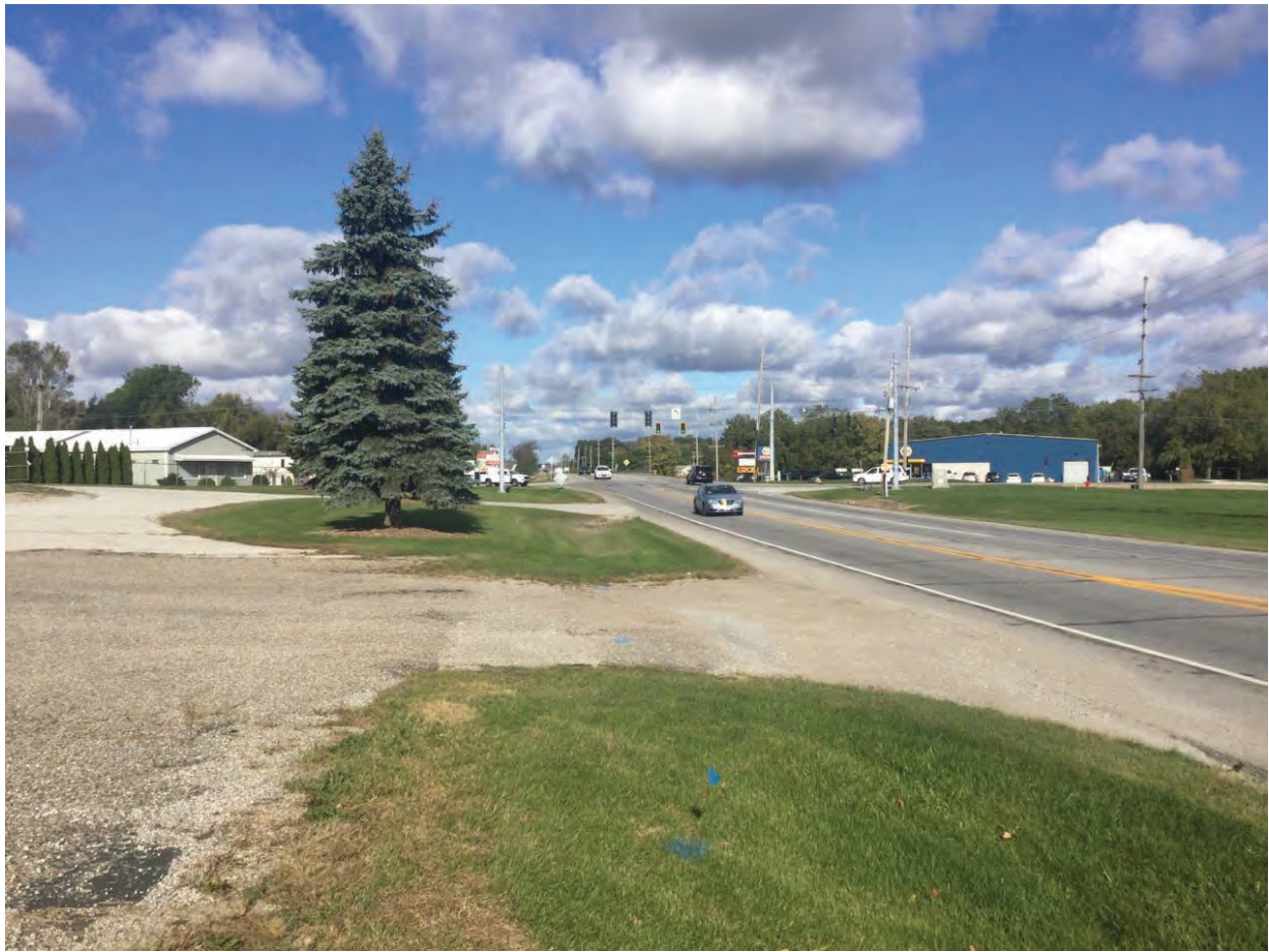
57. Looking north west along roadside US 20
