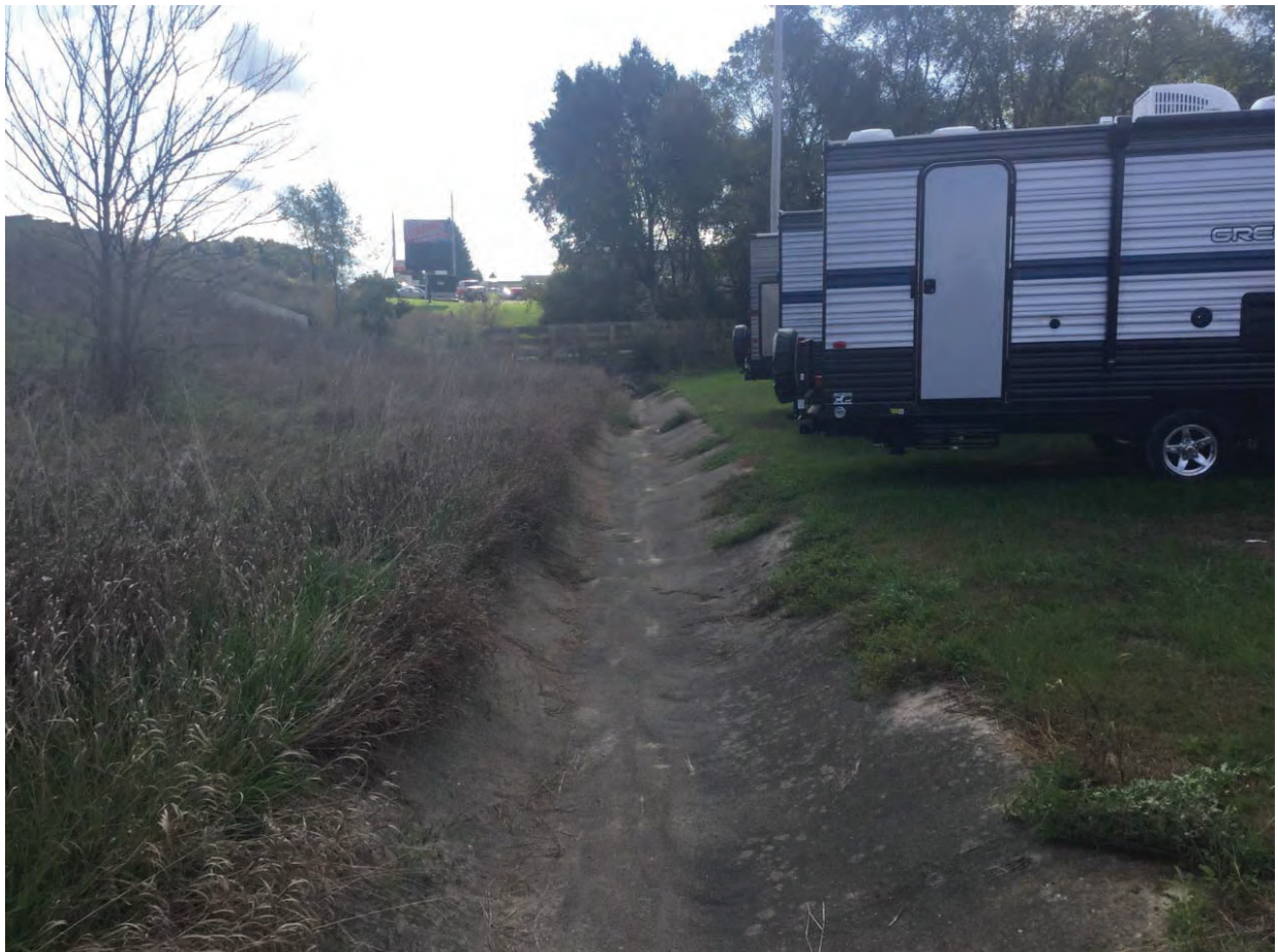
66. Looking south west at concrete side ditch
