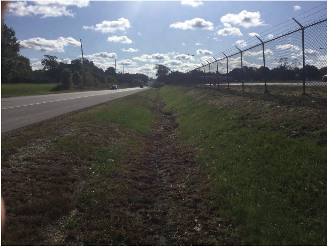
73. Looking southeast along roadside US 20
