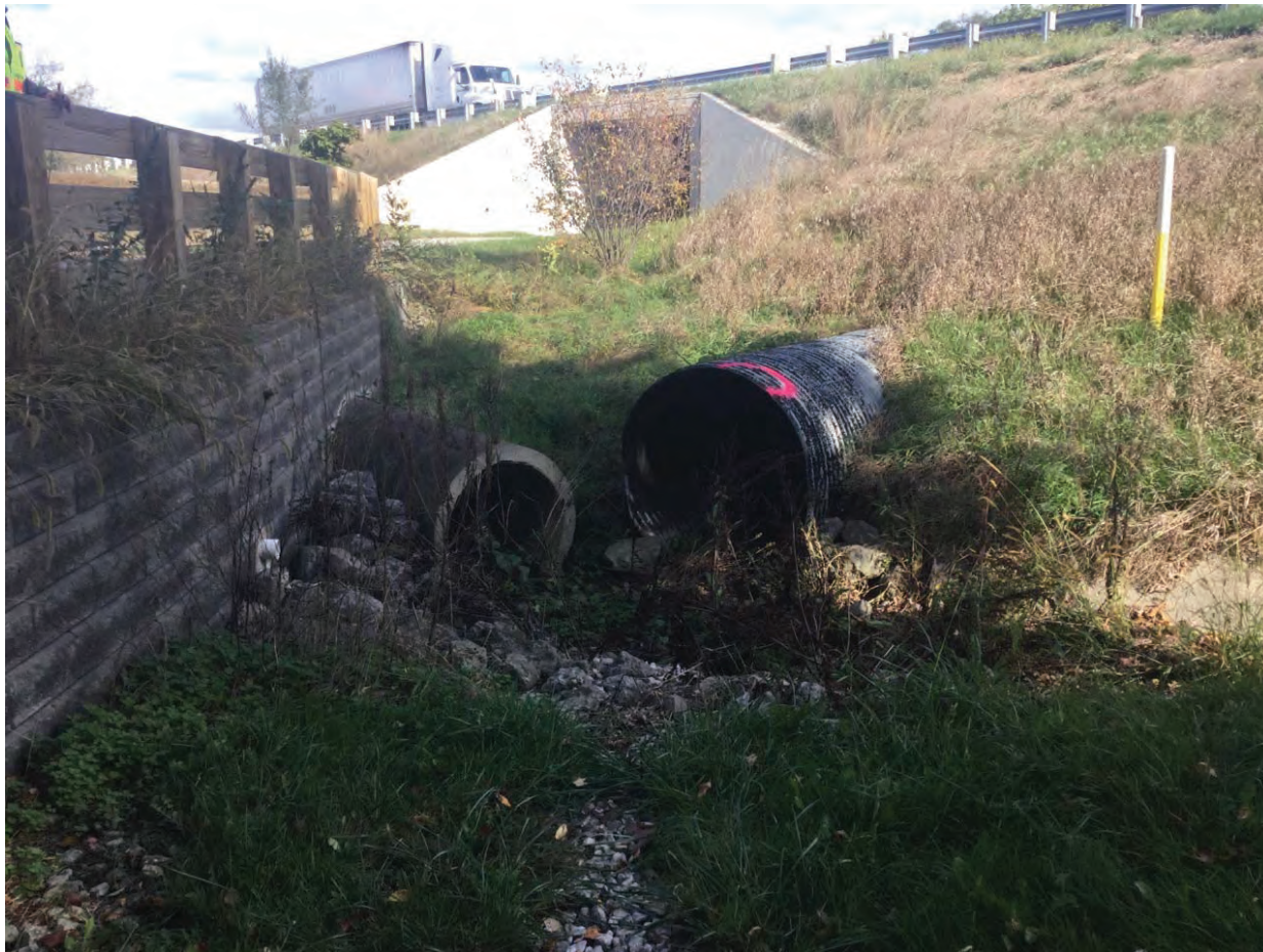
63. Looking north at Culverts along side Pumpkinvine Trail
