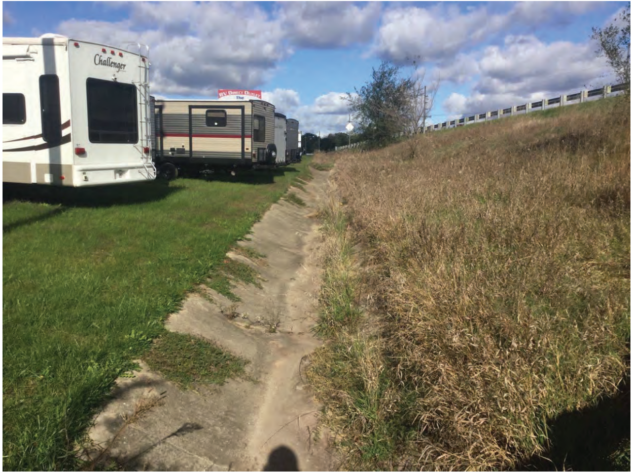
65. Looking north west at concrete side ditch
