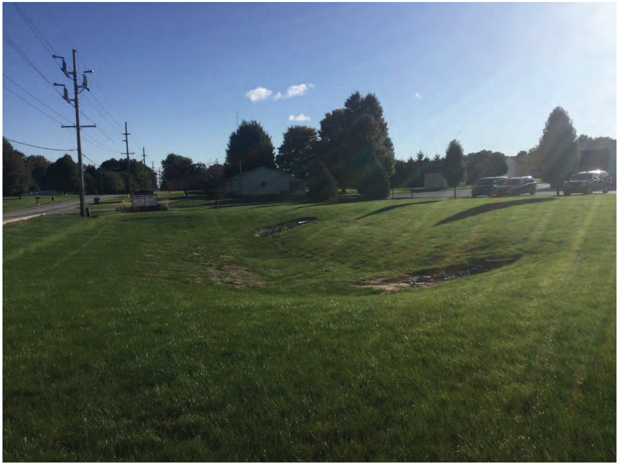
33. Looking east at retention area
